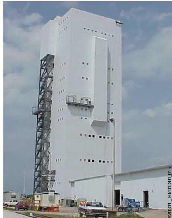
Figure 5.1.3.1-1 Vertical Integration Facility
