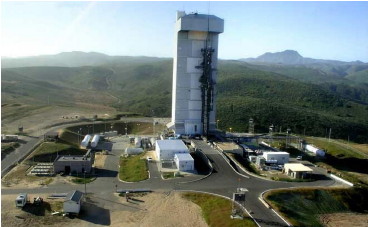
Figure 5.2.3-1 Space Launch Complex-3E
