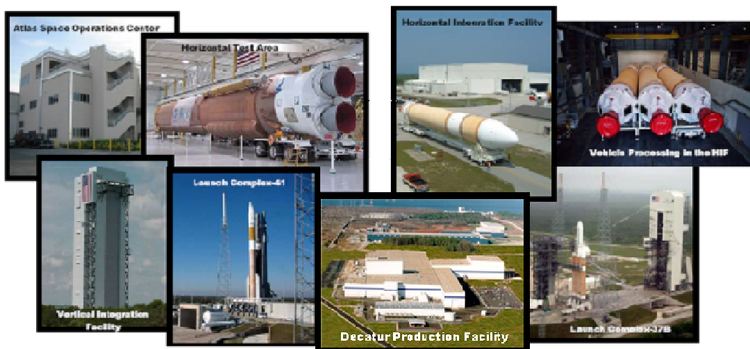
Figure 4: ULA Ground Infrastructure Assets 6
