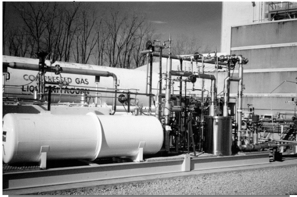
Figure 6. Boeing Liquid Hydrogen Densifier, Developed as Part of the X-33 Program
