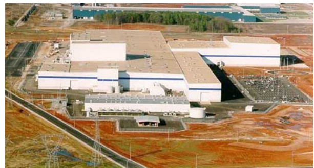
Figure 3. The 1.5-M-ft 2 State-of-the-Art Delta Manufacturing Facility in Decatur, Alabama
