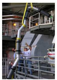
Fig. 8: Tail Service Mast (TSM) main structure and Fig. 9: Vacuum Jacketed Fill/Drain Line Installation
