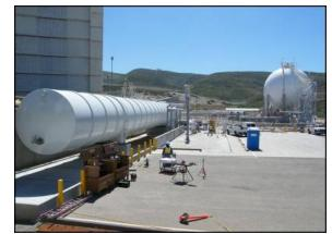
Fig. 10: The Cylindrical Auxiliary LOX Tank in Position
