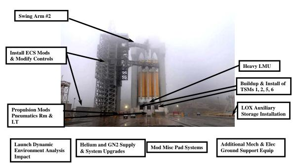
Fig. 7: SLC-6 Heavy Launch Vehicle (HLV) Modification Overview
