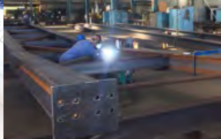
Off-Site Fabrication of MLP Underway
